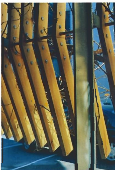
Above: The screen provides a visual connection to its heritage surroundings. Middle: The top of the entry screen provides the balcony handrail. Bottom: Detail of the celery top pine screen.
