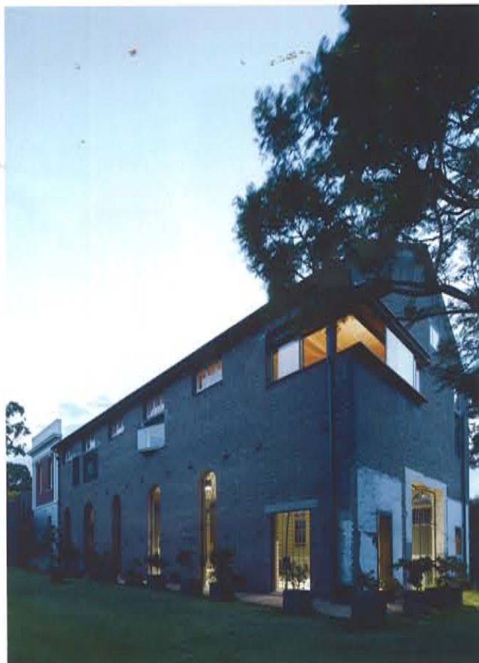
View of the north-eastern corner of the building from the garden.
