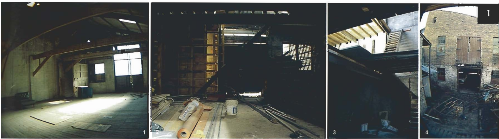
1-4 EXISTING AND MID-CONSTRUCTION VIEWS
