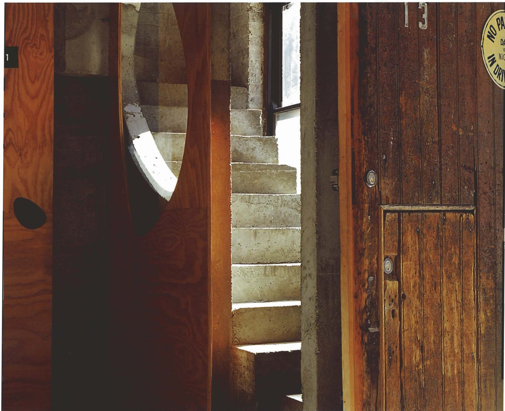
THE FREE-FORM SLIDING DOOR FRAMES THE IN-SITU CONCRETE STAIRS
