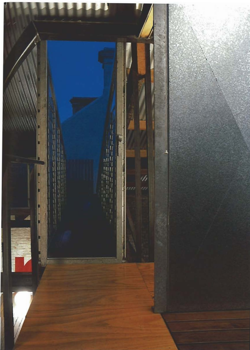
GALVANISED SHEETING WALLS OF THE BATHROOM
