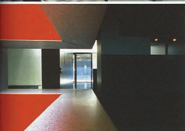
A striking light shaft is lined in red stained plywood.
