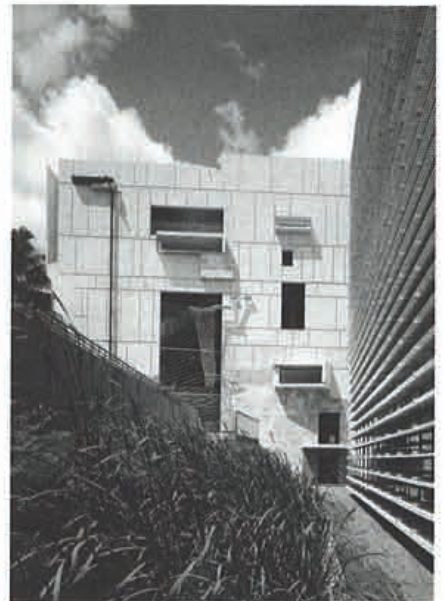
Neville Bonner Building, Brisbane, Queensland, 1998. Architekten: Donovan Hill
