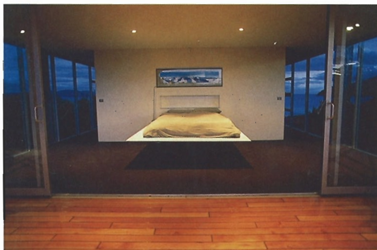
The bed is a steel structure bracketed off the core wall and cantilevered toward the centre of the room.
