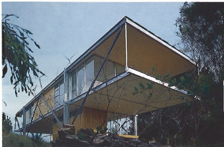
The floor and ceiling planes are extended beyond the building envelope to form covered decks.
