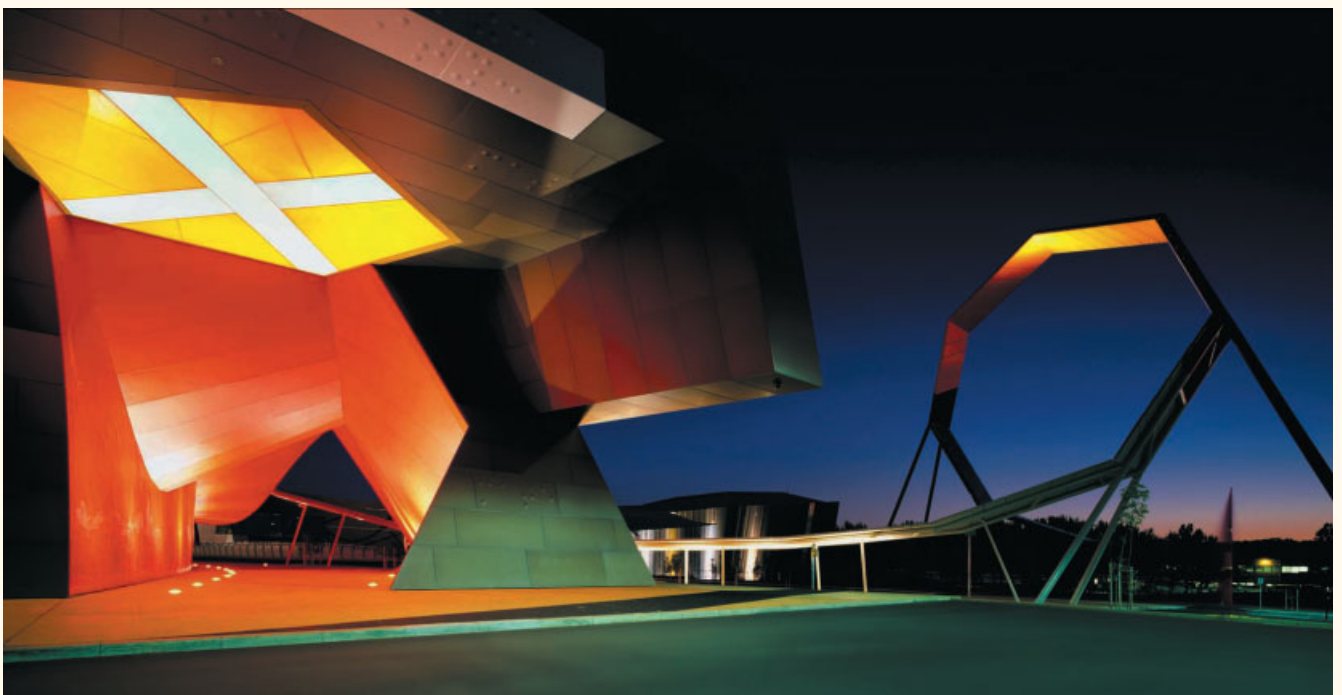
ARM, National Museum of Australia, Canberra, 2003 While the skin of the building and its plan comment on the past, a Boolean stream penetrates the building, setting up a dialogue with the more multicultural present, and thus embracing the future optimistically.
